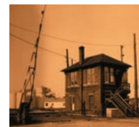
In Racine, Wis., this interlocking also controlled a set of gates. Rell Barrett Photo
