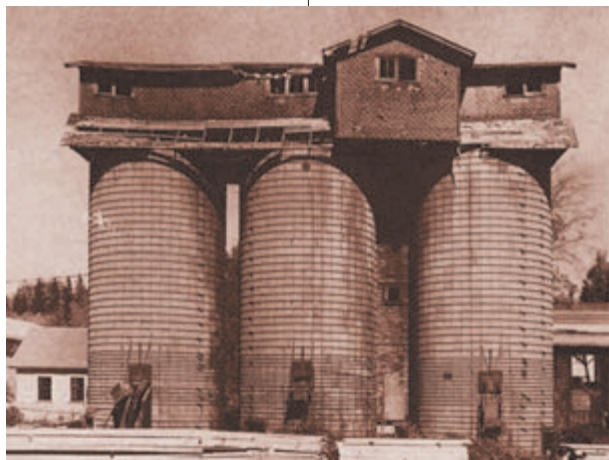
Bunker style coal silos were all a little different. This facility had banded wood silos and wooden roof. Prototype photos courtesy Railroad Model Craftsman Magazine.
