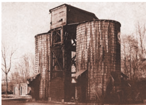
Bunkers at smaller dealers required less capacity. This two-silo facility in New York featured concrete slabs with metal band reinforcements.
