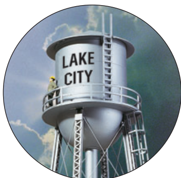
Detail of the City Water Tower tank, silver with black lettering.
